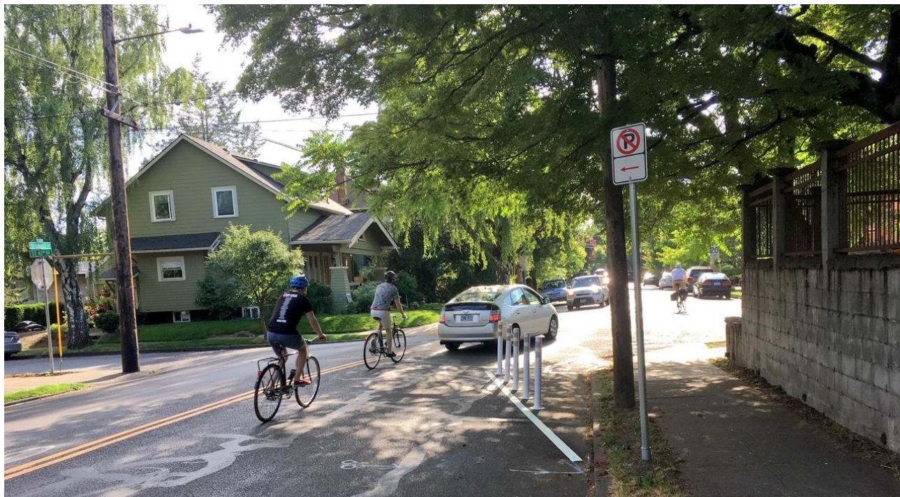
Flex-post serve as a traffic calming feature by temporarily reducing the vehicular lane width and restricting right-turn conflicts with bicyclists
