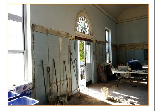
**Existing Vestibule** demolished and to be reconstructed to meet current accessibility requirements
