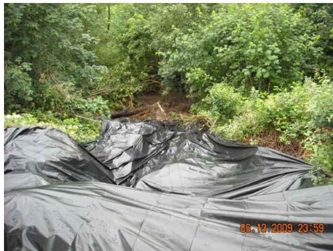
View looking down slope failure. Covered due to potential precipitation.
