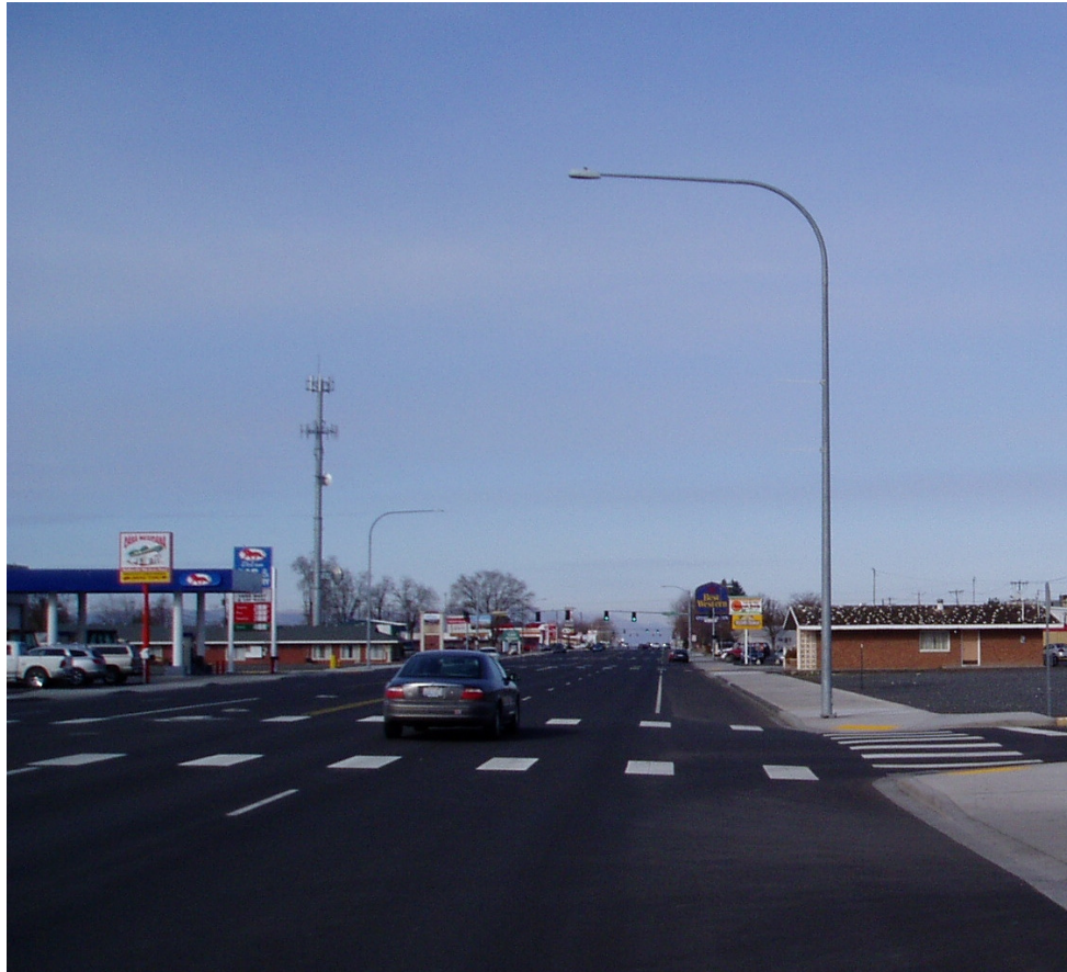
Fig. 4 - Typical modern-style galvanized metal arterial light
