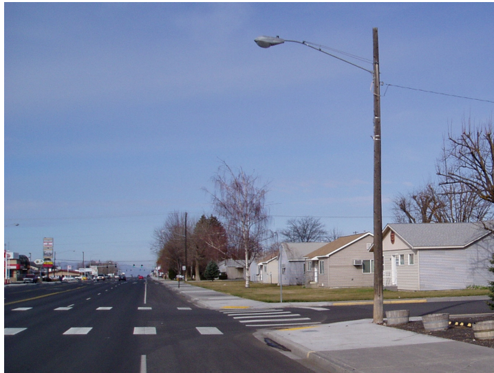
Fig. 14 - Wood pole with projecting light arm
