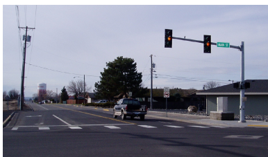
Fig. 1 - Typical modern style metal signal poles
