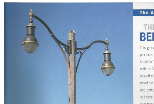
Scroll arm luminaire supports.
