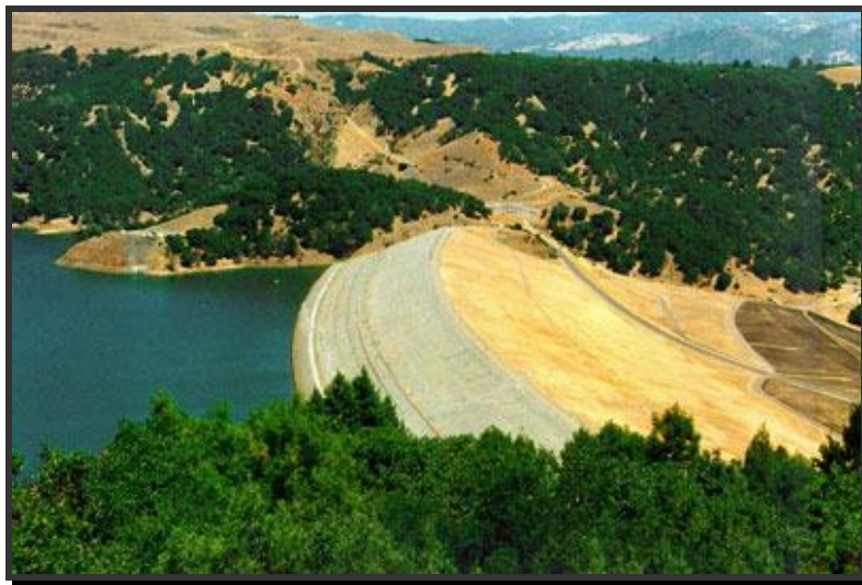
Photograph 1: Warm Springs Dam.
