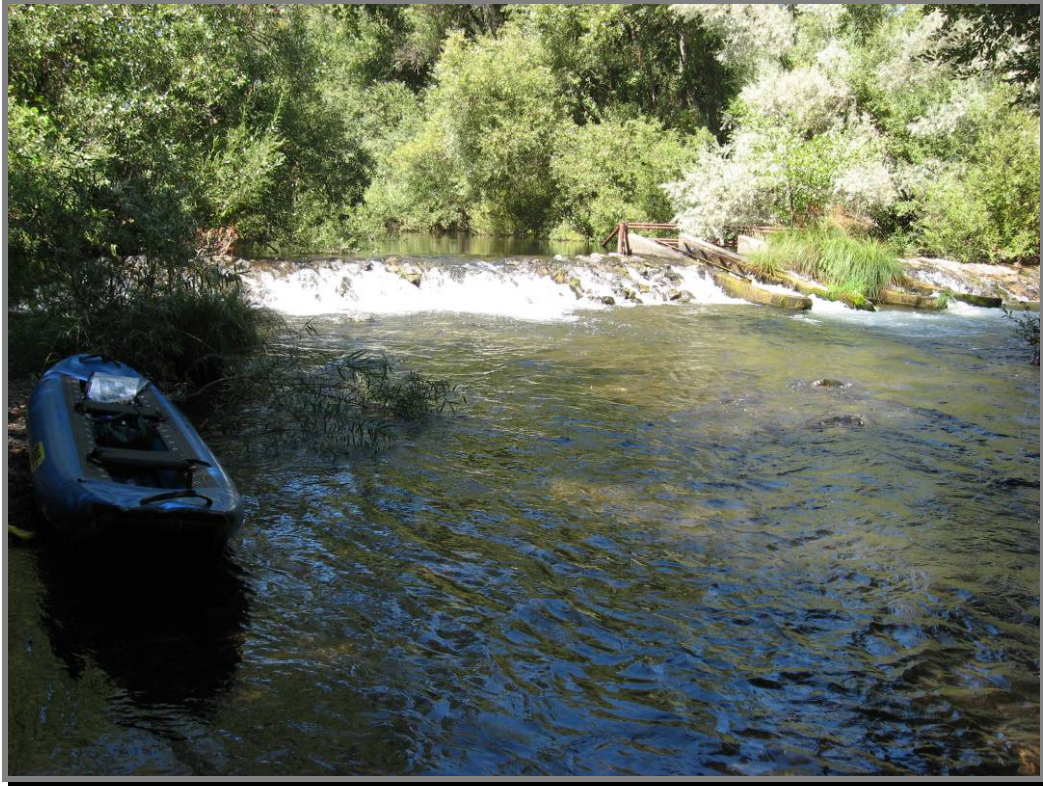
Photograph 8: Grade control sill, with fish ladder at top right, RM 3.2.
