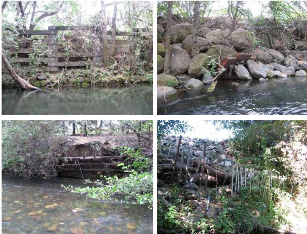
Figure 40: Bank stabilization features. (upper left) Board Fence, (upper right) boulder riprap with car parts, (lower left) a truck bed, (lower right) metal poles with logs and rocks.
