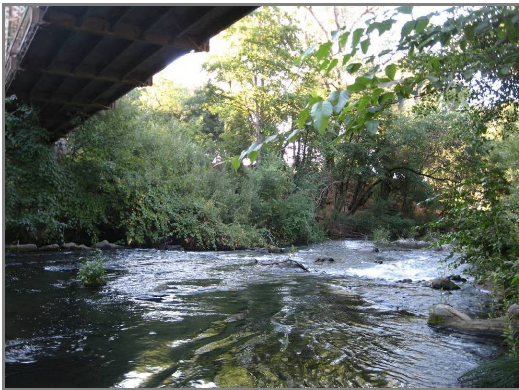
Photograph 7: Bedrock outcrop beneath Lambert Bridge, RM 6.6.
