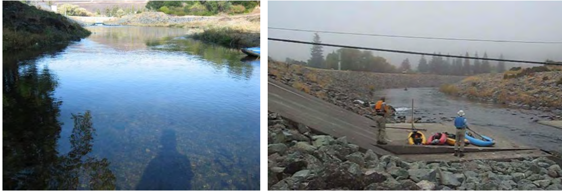
Figure 78: (left) looking upstream at the deep pool downstream of the measuring flume structure, (right) preparing to launch from the measuring flume structure.
