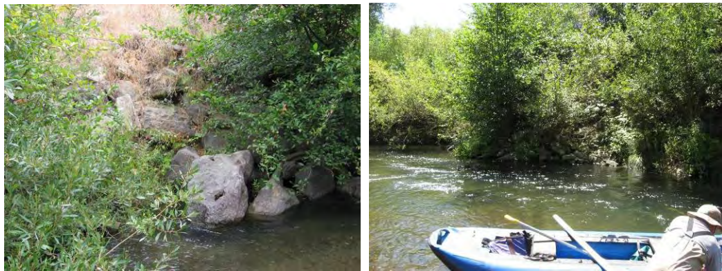
Figure 7: (left) Boulder riprap along streambanks, (right) a pool with riprap along the right bank.
