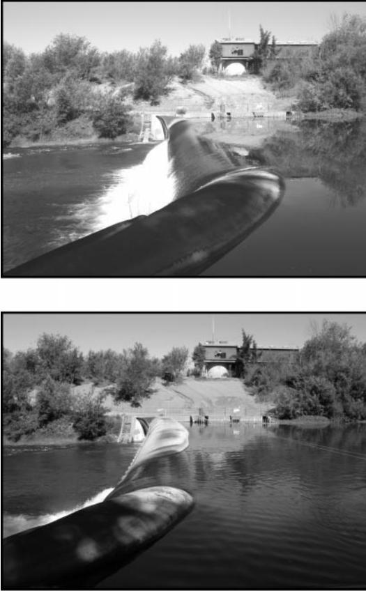
FIGURE 2.—Photographs of Mirabel Dam on the Russian River, California. The dam is shown in its normal inflated configuration (top panel) and in a notched configuration (bottom panel).
