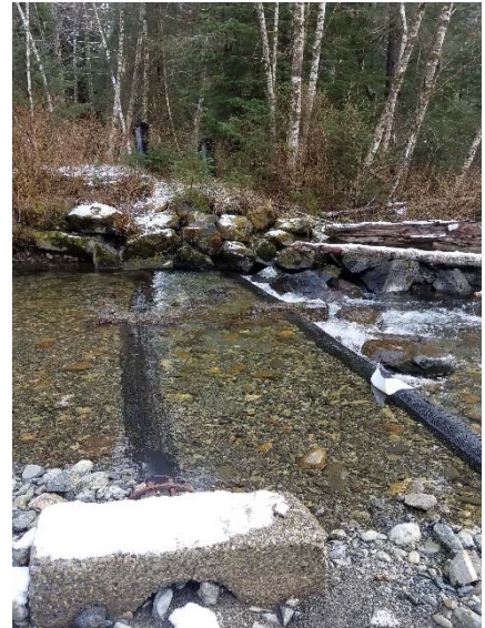
Photo 12 - Existing Perforated Pipe Intake
