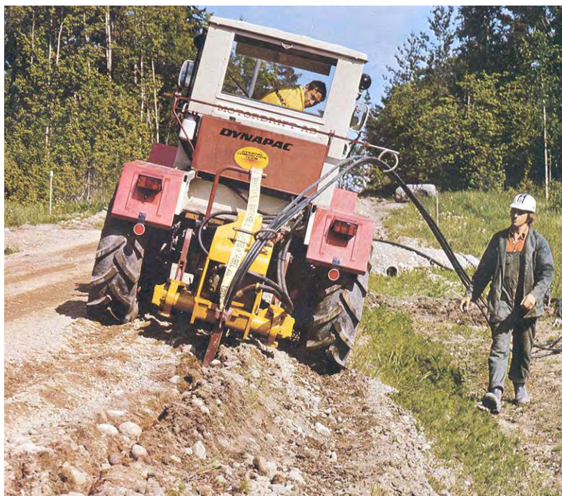
Figure 13 Installation of DC cable by direct burial
