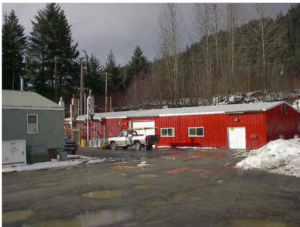
Photo B-8 – THREA powerhouse in Hoonah.
