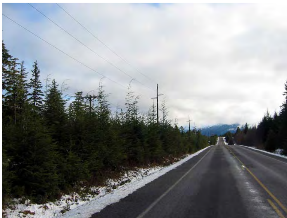
Photo B-14 – Mitkof Highway south of Petersburg with 138-kV Tyee transmission line to the left.
