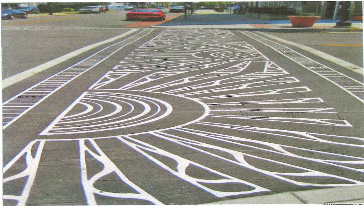
Figure 4.18 – Photograph of a Designer Crosswalk in Ocean City, New Jersey
