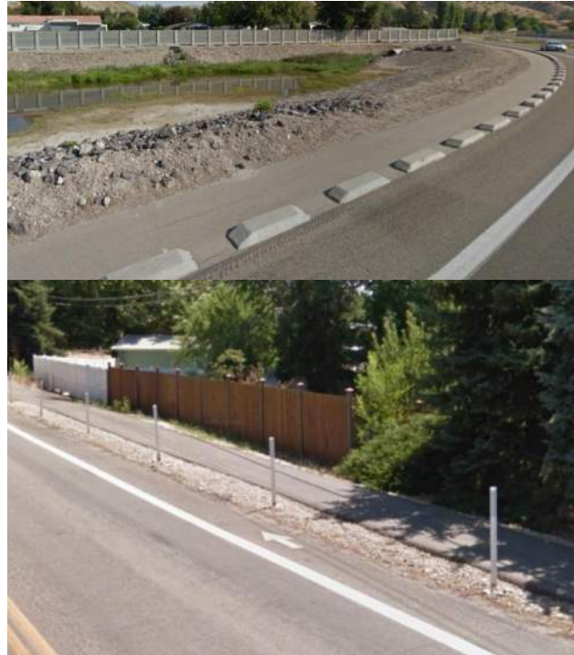
Extruded curb and flexpost separated walkway sections on Hill Road (Boise, ID) Images Source: Google Streetview
