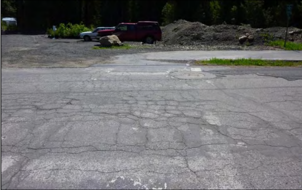
Figure 4 – Existing Pathway Crossing Marking (June 16, 2011), repainted summer of 2011
