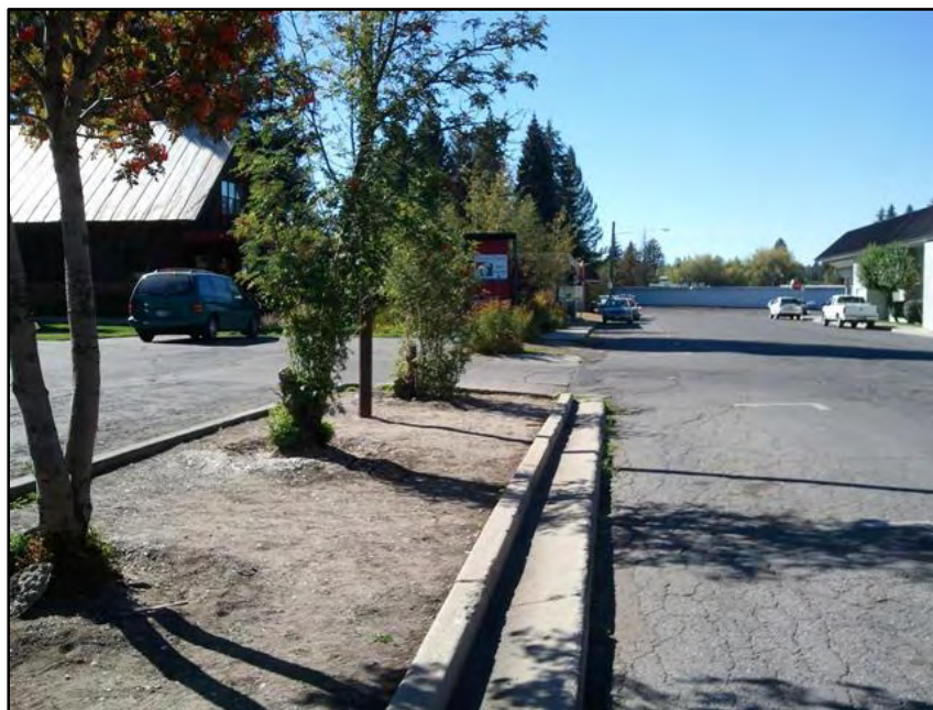
Figure 26 – Existing missing sidewalk connection in downtown McCall
