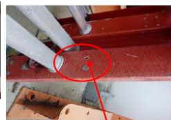
Missing Rivet
